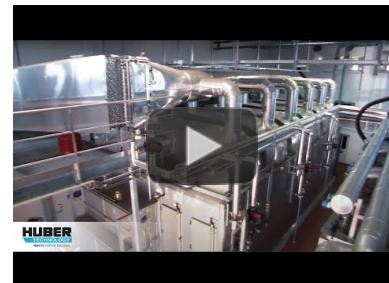
Video: HUBER Belt Dryer BT for medium temperature sewage sludge drying
