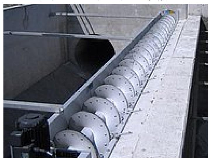
**Storm screens** are provided to retain solids at combined sewer overflows and reduce surface water pollution. Their power consumption is very low since they operate only periodically (See HUBER Storm Screens).
